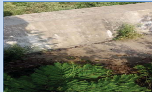
Name of the project: Murlinagar Name of the district: Rangareddy Incomplete check dam – Non construction of apron, etc.
